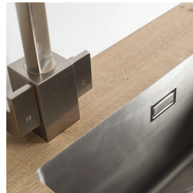
These images show a stainless steel sink fitted flush to the custom-made surface. The joint is completely waterproof, making it brilliantly hygienic and easy to clean.
