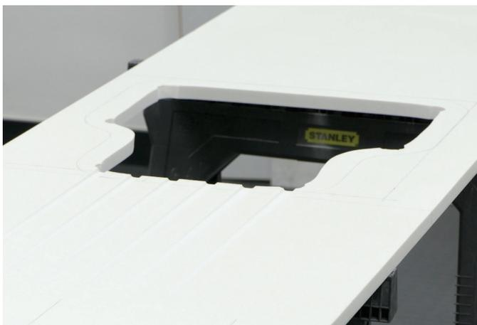
Once the adhesive has set, using a two-flute bottom bearing guide cutter, set the bearing so that it is contacting the uppermost inner face of the sink. Trim the excess material. Apply a rounded profile around the top edge of the sink. Finish the raw edge as described in the section 'Surface Finishing'.
