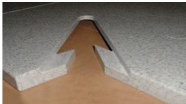
(9) Remove template, counter is now ready
