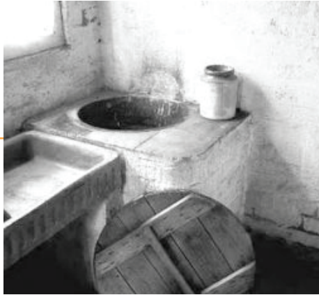
1908 Edwardian houses were built with a 'Copper' the only means of obtaining hot water in significant amounts.
